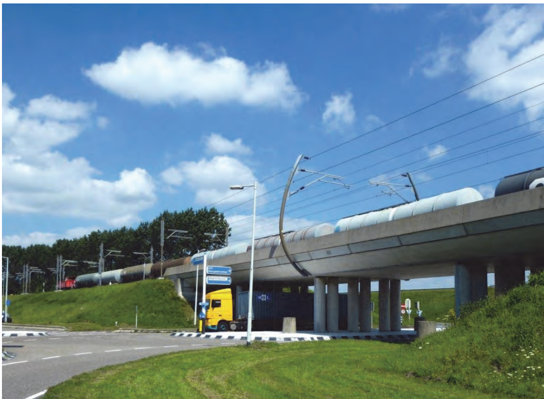
Harbourline near Botlek handover station.
