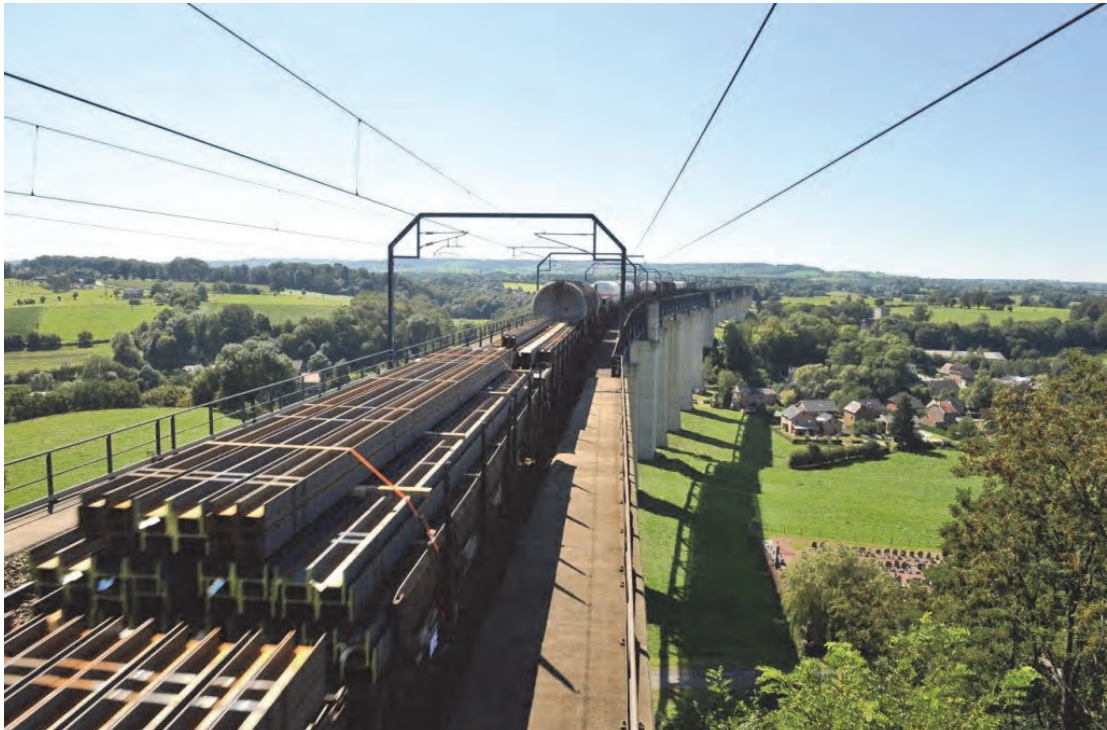
Viaduct of Moresnet on the Montzenroute.
