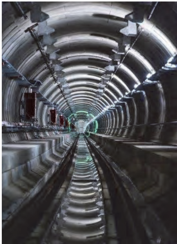
The Liefkenshoektunnel between the right and the left bank of the port of Antwerp was inaugurated in December 2014 Infrabel – Herchaft Eric – Reporters
