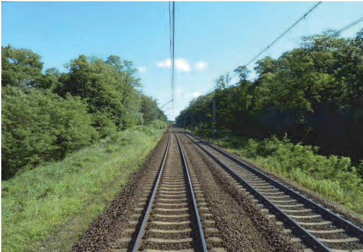
Line between the operating bridge on Odra river and Rzepin Source: DB Netz AG
