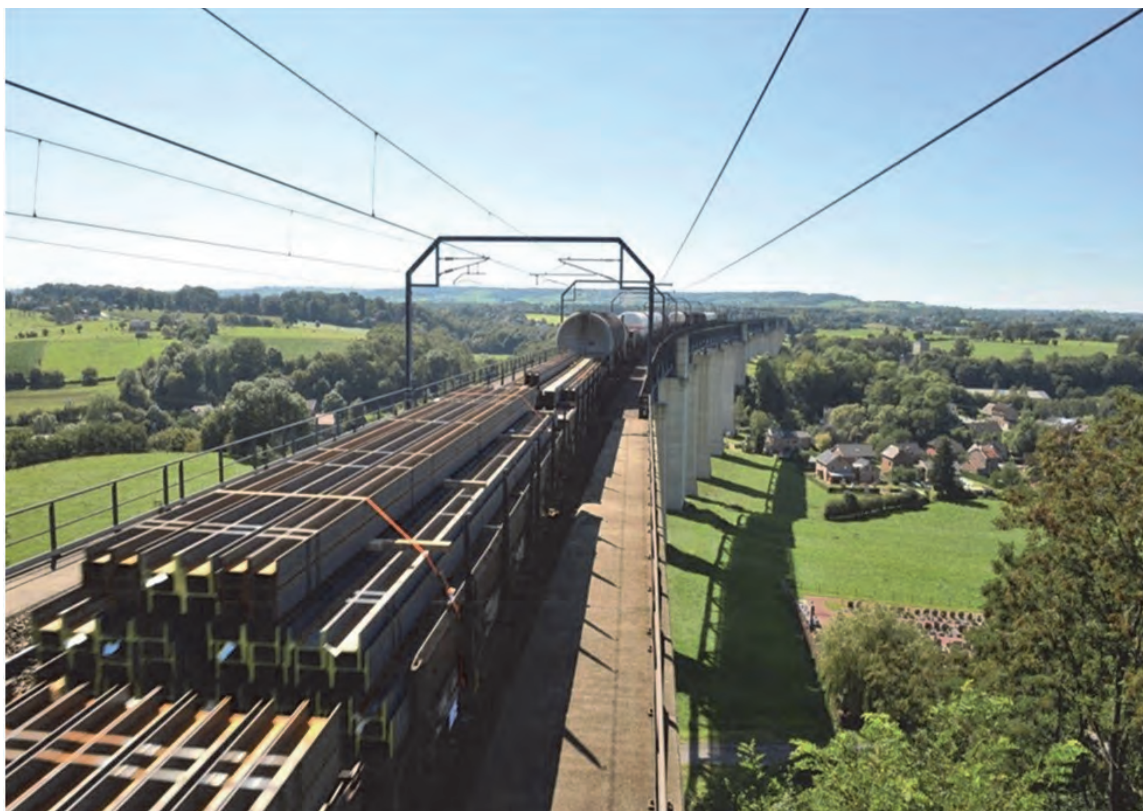
Viaduct of Moresnet on the Montzenroute Photographer: Johan Dehon. Rights: Infrabel
