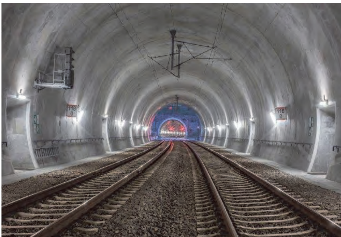
New tunnels for combined transport Archive SŽDC
