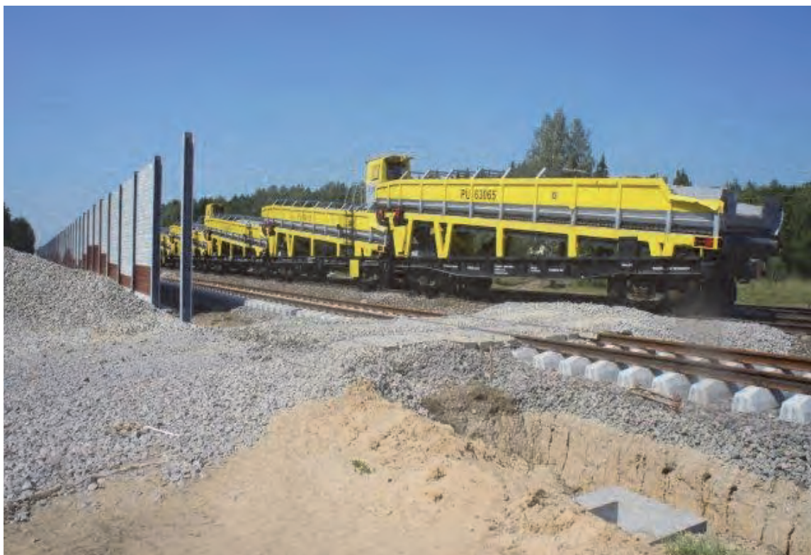
Building of the new Rail Baltica line Source & Copyright: Lietuvos Geležinkeliai
