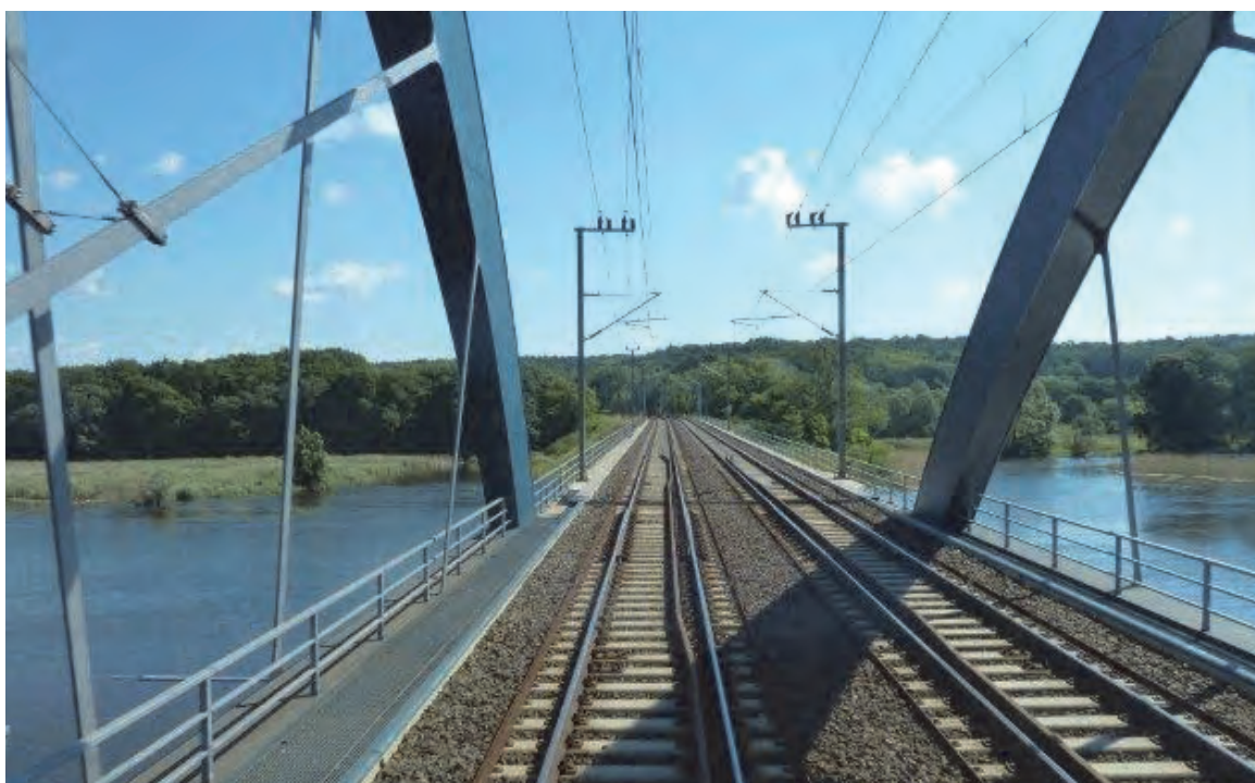
Bridge over Odra river Source: DB Netz AG
